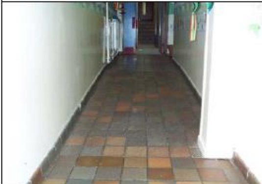
Photograph 3 Ramped floor on the lower ground floor.
